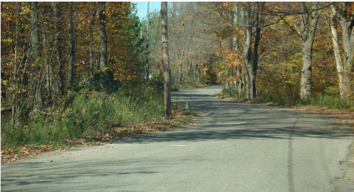
Photo 8-56: Right-of-way and horizontal alignment along Milborough Line between Concession 11E and Derry Road
